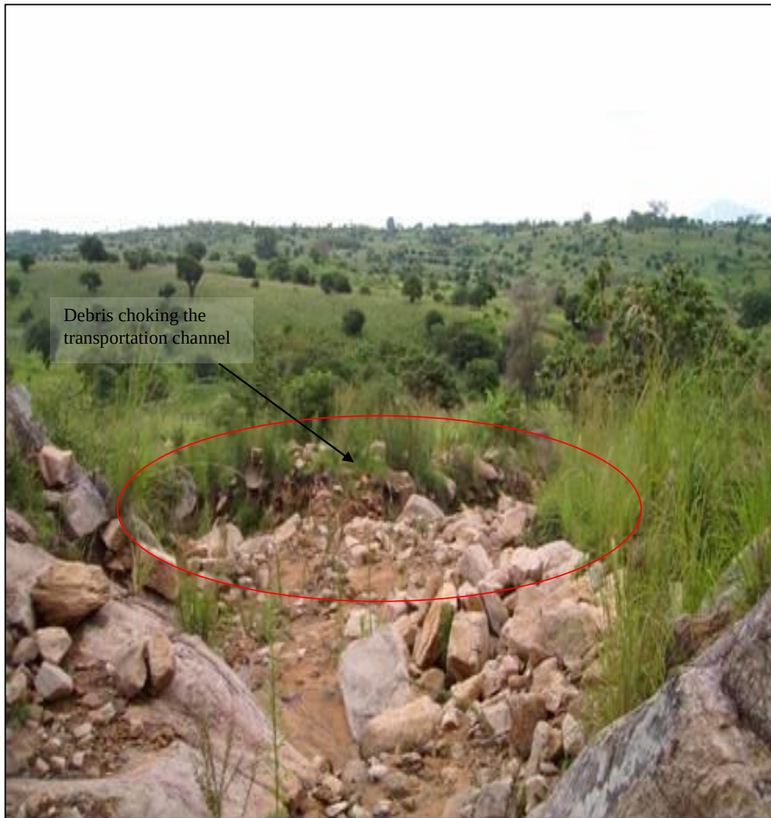
Plate 8. Debris Deposited in the Transportation Channel.
